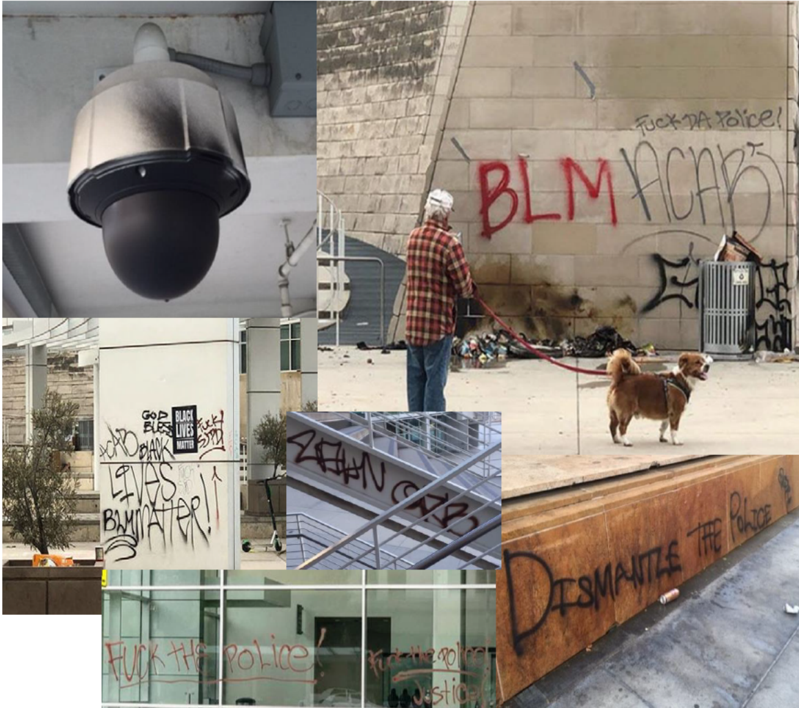
Figure 64. Some of the Extensive Vandalism at San Jose City Hall
